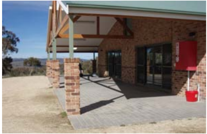
Photo: Exit from dining room & step
