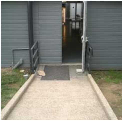
Photo: Rear exit from Dining Hall to paved path to carpark
