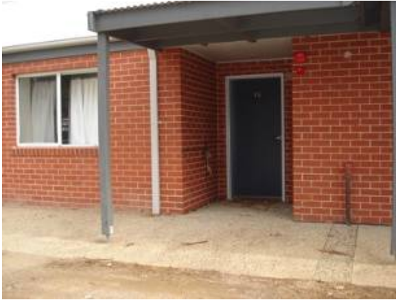
Photo: Room 15 Entry & Internal corridor
