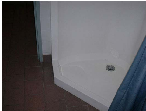
Picture 4. Shower access
