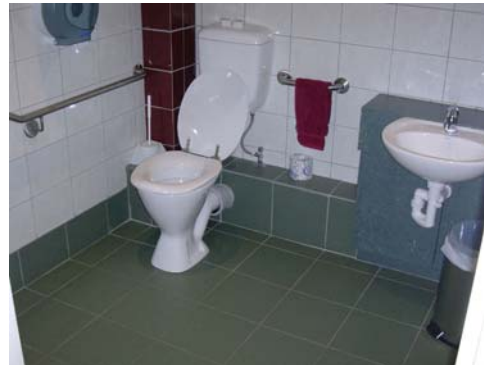
Picture 6. Accessible toilet
