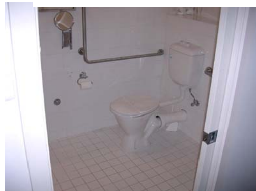
Picture 13: Toilet room No 12
