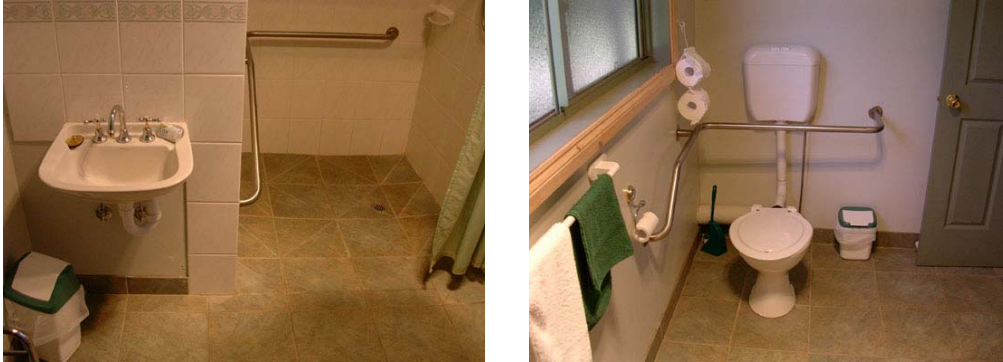
Pictures 8 & 9. Shower and toilet
