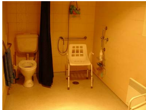
Picture 11: Right side bathroom
