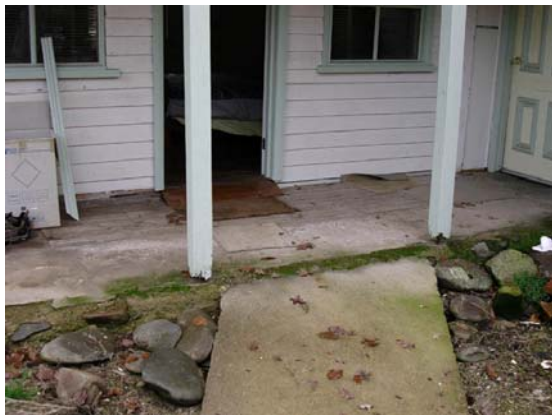
Picture 8: Entrance Cottage bedroom
