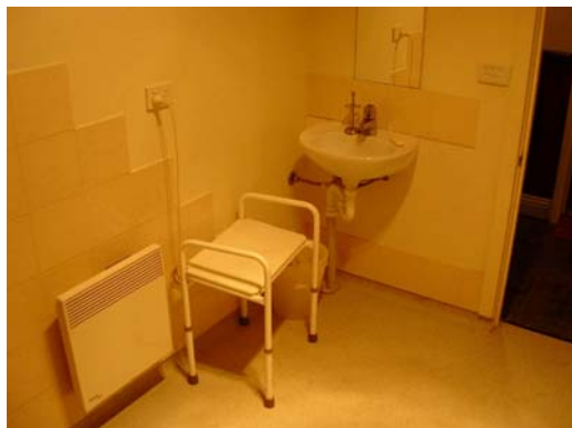
Picture 10: Right side bathroom
