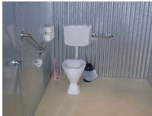
Picture 5. Accessible toilet
