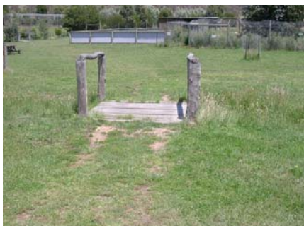
Picture 12: Another of the smaller bridges.
