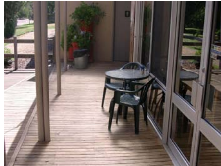
Picture 5. Path of travel to accessible toilet
