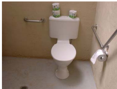
Picture 4. Accessible toilet
