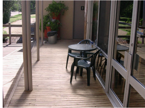
Picture 3. Path of travel to accessible toilet
