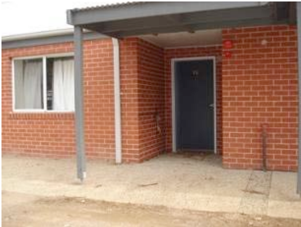
Photo: Room 15 Entry & Internal corridor
